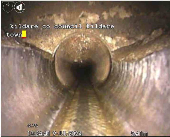
Melitta RdX_20082024_1649_Sec1_Insp1_MH_0m.jpg, 00:00:00, 0.00 m Start node, manhole, reference: Melitta Rd
