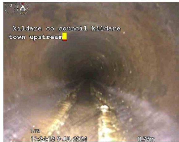
Line AX_8e3d9872-70a6-485c-b95d-df6be60fe84c_20240820_171 948_311.jpg, 00:01:57, 0.00 m Water level, 5% of the vertical dimension, Unable to determind distance
